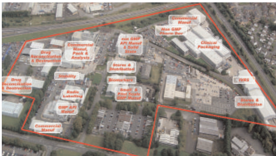
Almac's UK headquarters site at Craigavon combines and integrates activities across the whole range of pharmaceutical discovery and development to commercial production.
